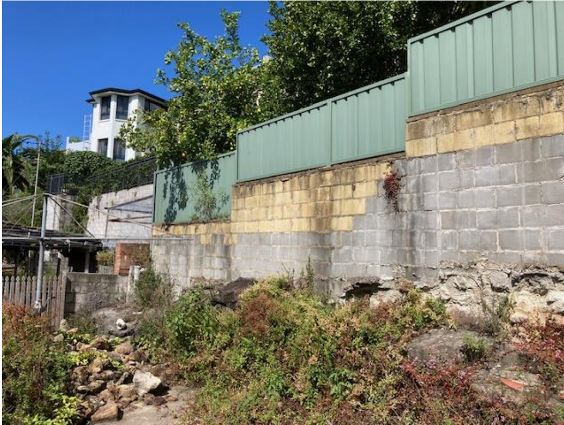
Photo 5 - Looking at sandstone bedrock and retaining walls supporting the rear southern boundary
